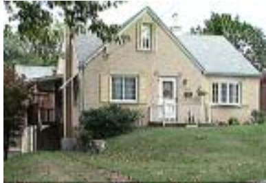
TCV's new MR house on Tioga Street
